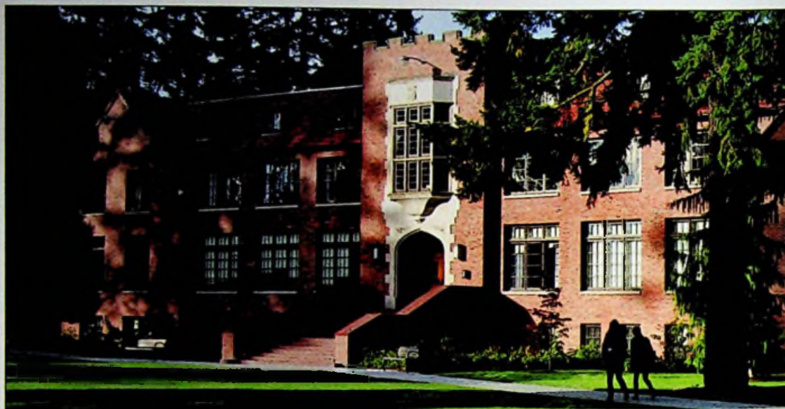
THE MUSIC BUILDING IS 60 Yup, the only Puget Sound classroom building that isn't named for a person opened in 1953. It was the third classroom building to be constructed on the campus, after Jones and Howarth halls, and we still delight in hearing piano scales coming through its open windows when walking through Karlen Quad on warm spring afternoons.
