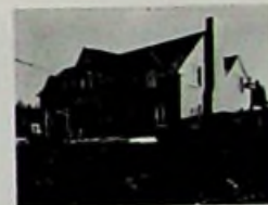
President's House under construction, 1950
